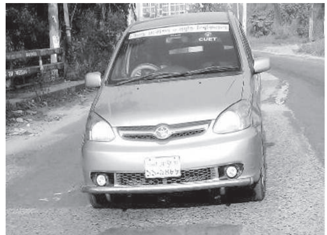
c) Very poor road pavement condition
