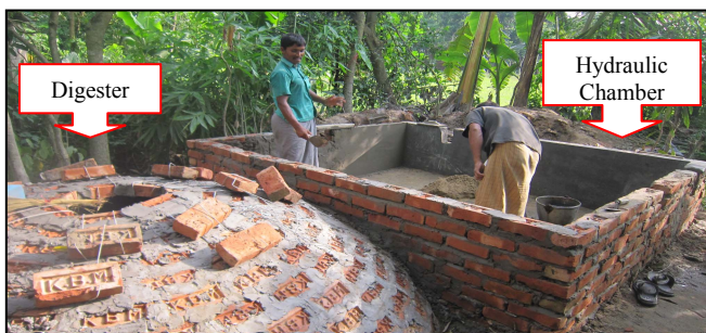
Fig. 7 The construction of outer structure of the digester and hydraulic chamber
