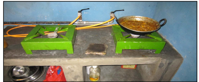
Fig.10 The stove burns and food is cooked using the gas produced by the system.
