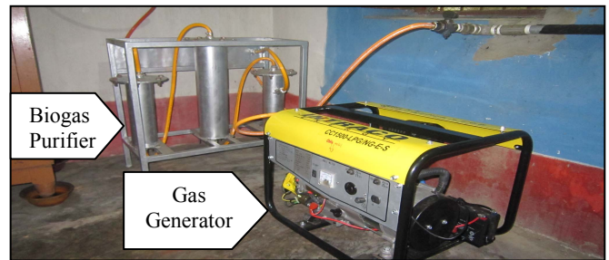
Fig. 11 The gas generator with the biogas purifier used in this system.
