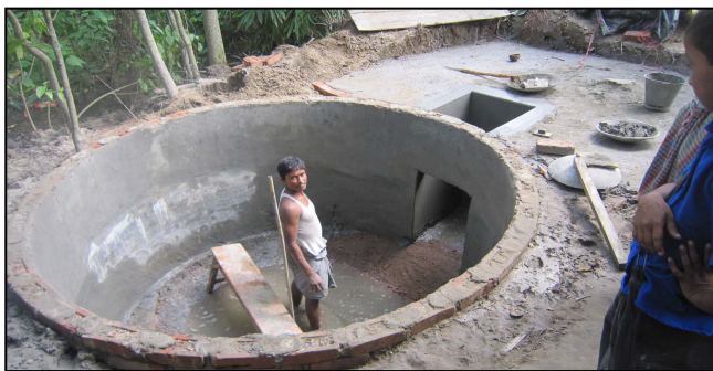
Fig. 6 The base construction of the digester and hydraulic chamber
