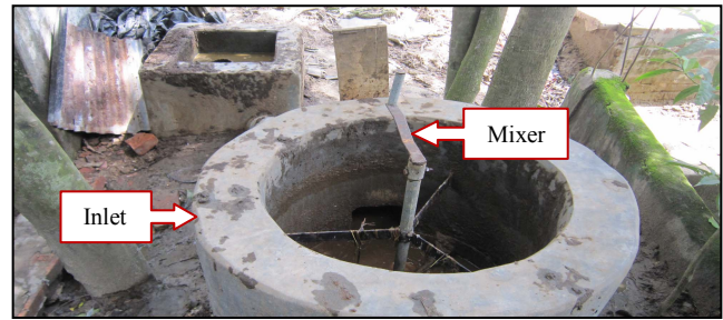
Fig. 8:- The Inlet of the system with mixer
