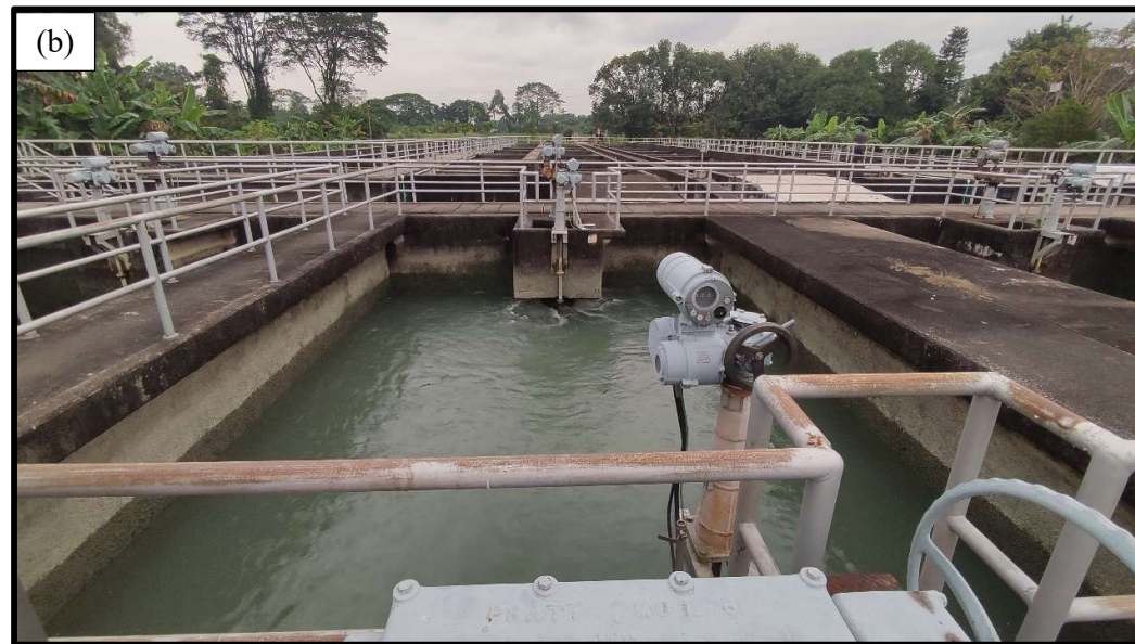
Figure 3.8 (a, b): Rapid gravity sand filters of MWTP (Source: Google Earth and CWASA)
