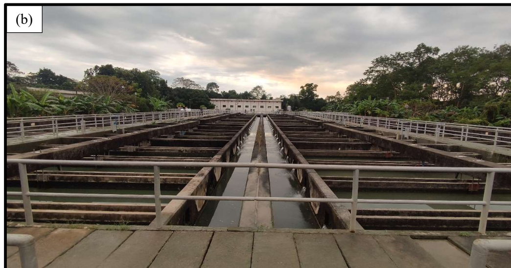
Figure 3.7 (a, b): Clarifiers of MWTP (Source: Google Earth and CWASA)
