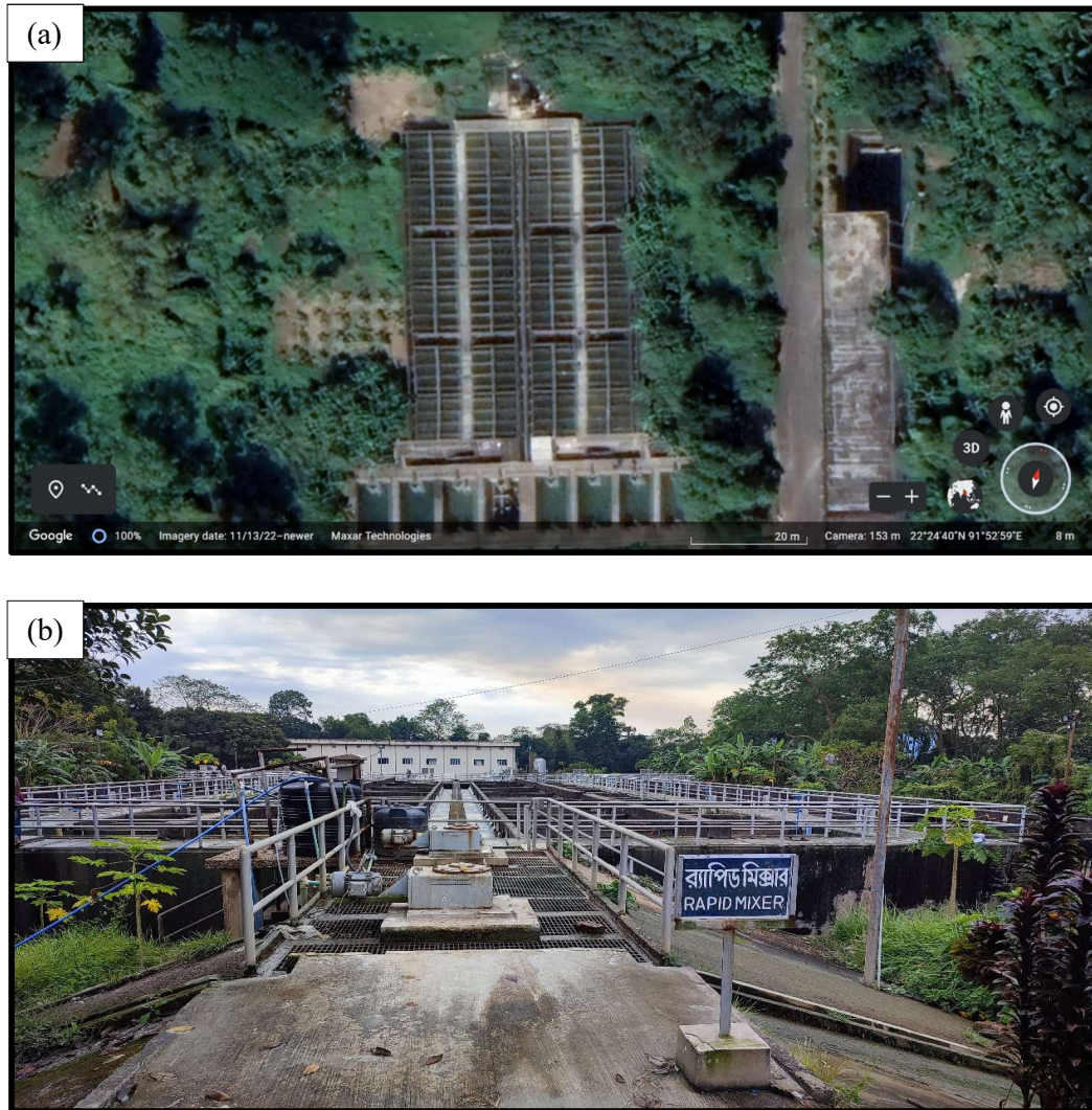
Figure 3.6 (a,b): Rapid mixing chamber of MWTP (Source: Google Earth and CWASA)
