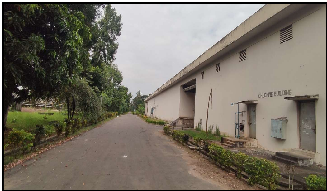
Figure 3.9: Chemical and Chlorine Building of MWTP (Source: CWASA)
