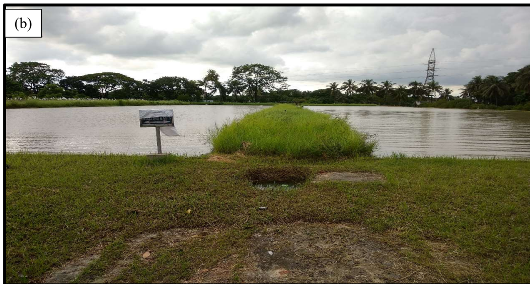
Figure 3.5 (a, b): Primary Sedimentation Basins of MWTP (Source: Google Earth and CWASA)
