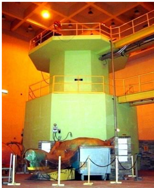
Fig. 3.7: Partial view of TRIGA Mark II research reactor at AERE.
