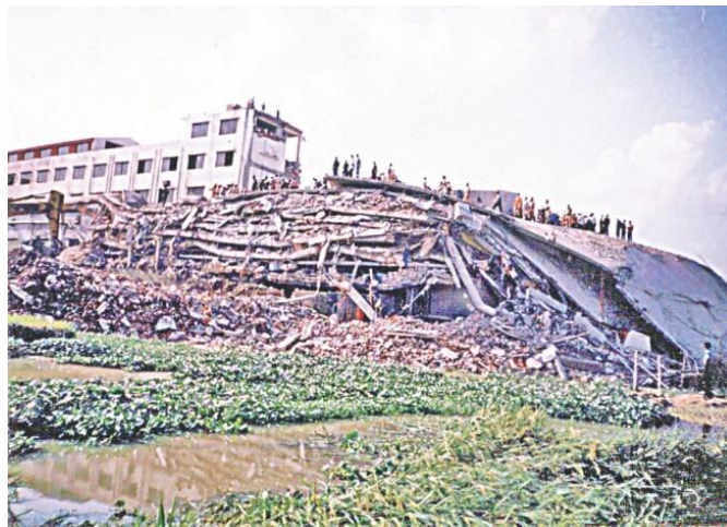
Figure 1.1: Under construction Garments factory collapsed in 2005 in Dhaka (IEB investigation Report, 2007)
