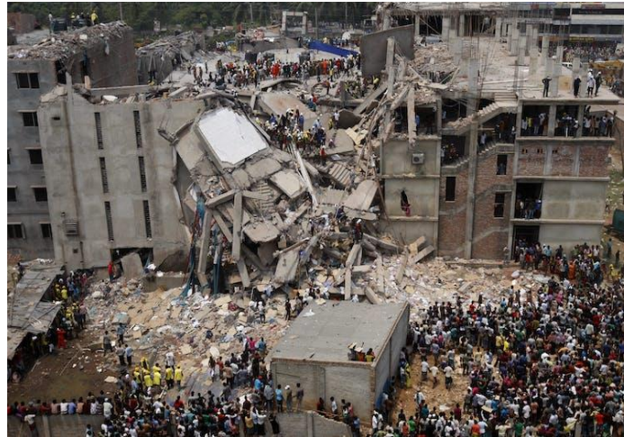
Figure1.2: Rana Plaza factory building collapse in 2013 at Savar, Dhaka
