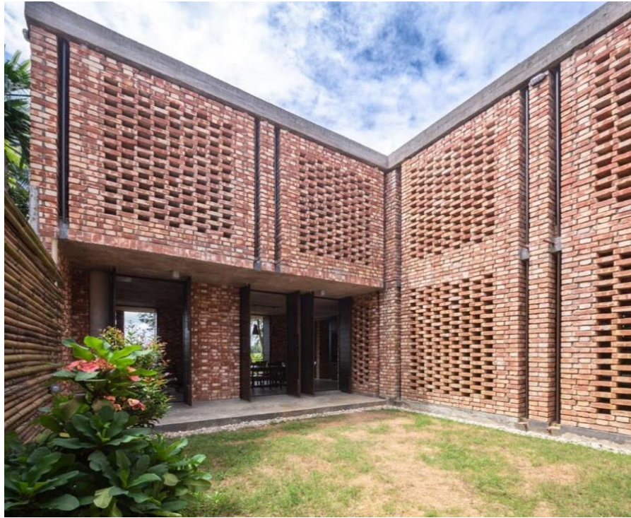
Figure 2.12: A view of masonry units in a building
