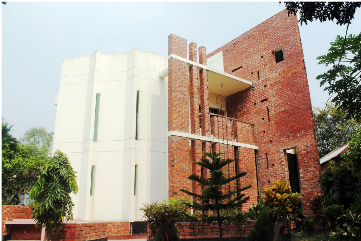
Figure 2.13: A view of masonry joints in a building
