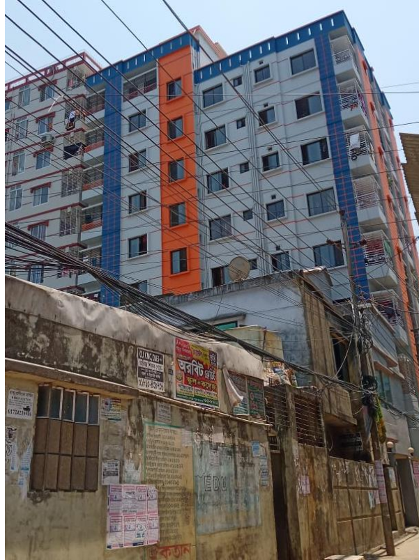
Figure 2.18: Pounding possibility due to adjacent building location
