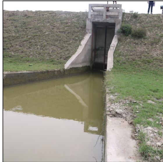
Fig. 3: Zialtola Sluice of Polder-26 (View from country side)
