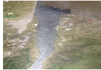
Fig.2:Site1(Barakuthi Mukta Mancha)
