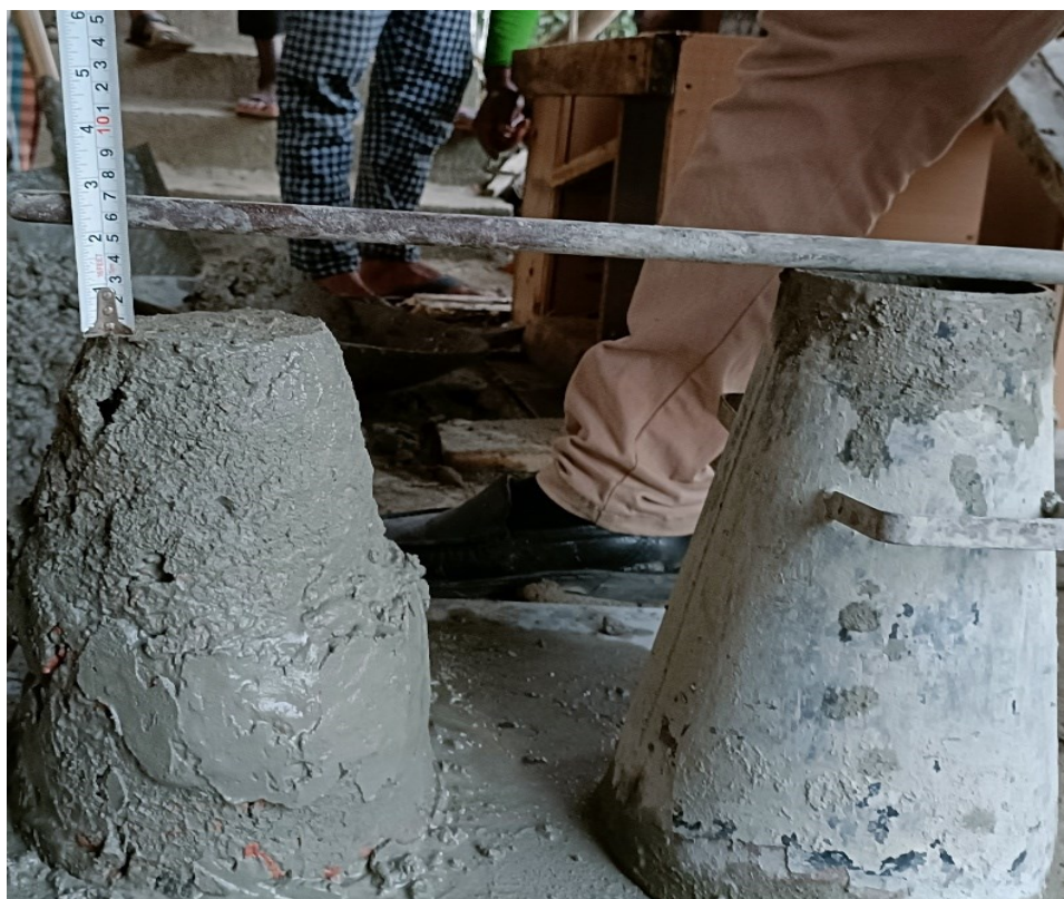
Fig. 3.28. Measuring of Slump During Slump Test While Concreting
