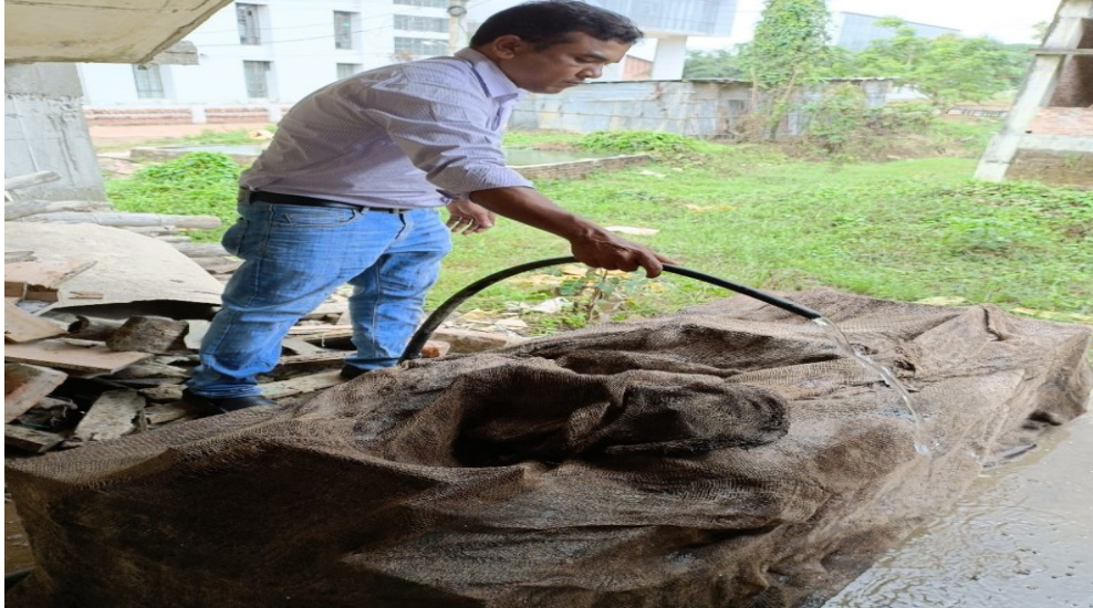
Fig. 3.29. 28 Days Water Curing Using Jute Jacketing
