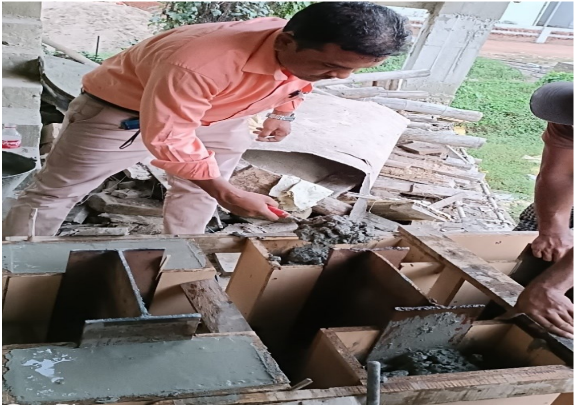
Fig. 3.25. Pouring of Concrete to the Mould of Specimen
