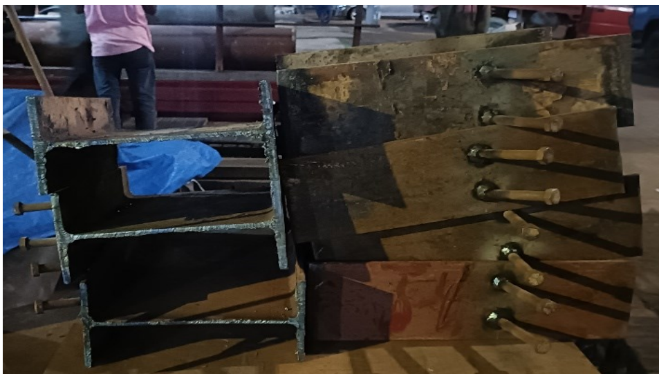
Fig. 3.17. Stacked Finished Piece of Girder after Completion of Welding
