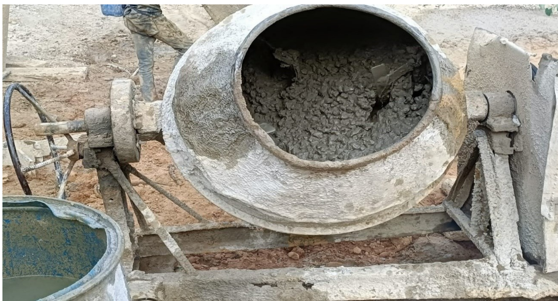
Fig. 3.24. Concrete Mixing Using Mechanical Concrete Mixture Machine
