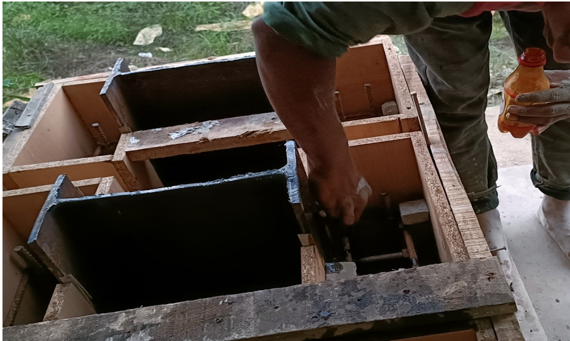
Fig. 3.23. Oiling on Formwork Before Casting
