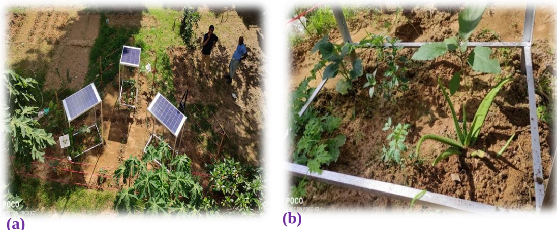
Fig. 3.10: (a) Implemented APV Project in EME Building premises, CUET (Top View), (b) Crops plantation under Solar Shade in APV system.
