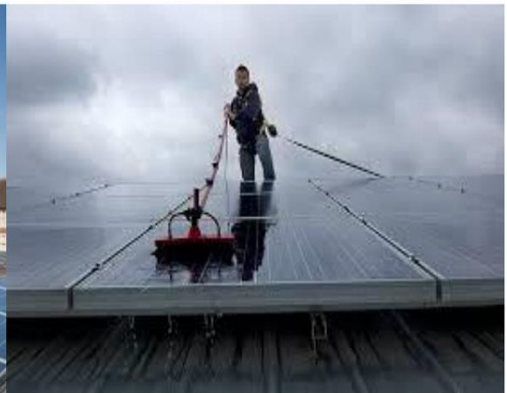
Fig. 4.3: Vacuum Suction Cleaning
